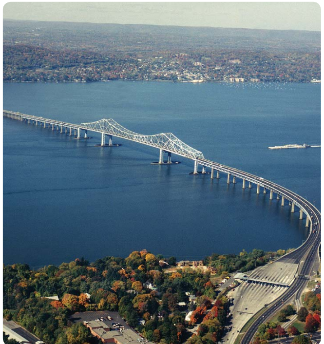
The Tappan Zee Bridge is an example of a project subject to the Environmental Impact Statement process.
