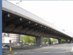
Modern steel bridge Hammersmith flyover, West London
