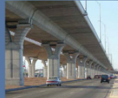
Modern concrete bridge U.S. Route 83, TX
