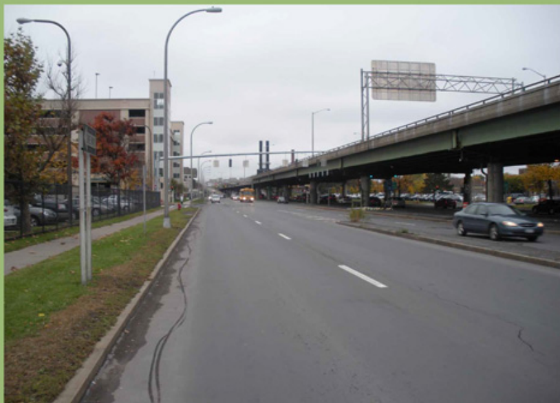
I-81 existing conditions, view south
