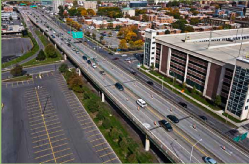
I-81 existing conditions, view north
